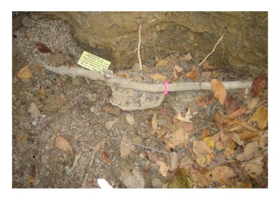
A typical lead service branch. By gently scraping the pipe where it enters the house you may be able to see whether you have copper, which will be copper colored, or lead, which will be dull gray (if you have galvanized iron, replace it before it starts leaking)
